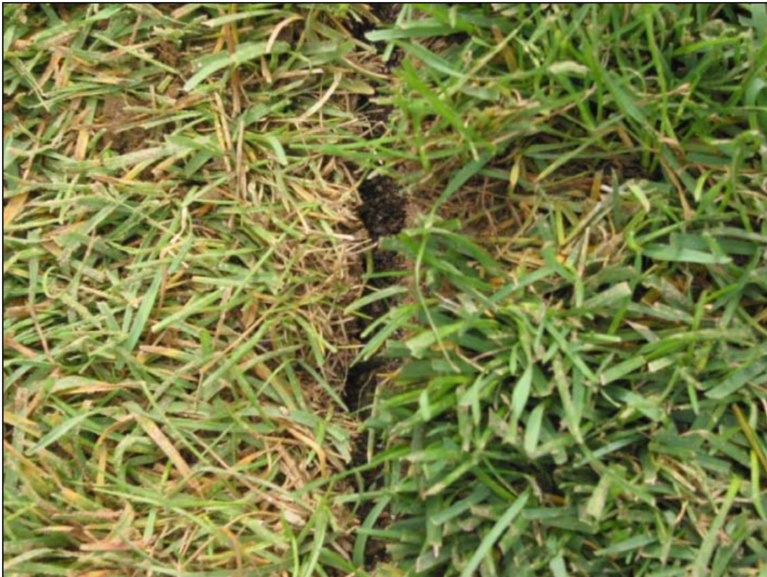
When laying sod, seams should be pulled tightly closed. Proper repair steps should be taken for seams that open after installation.
