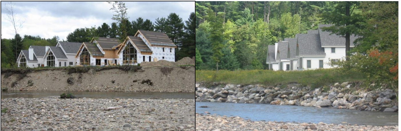
Development built next to river on lands not in the NFIP designated flood hazard area, where rip-rap used to protect the investment began failing after seven years.
