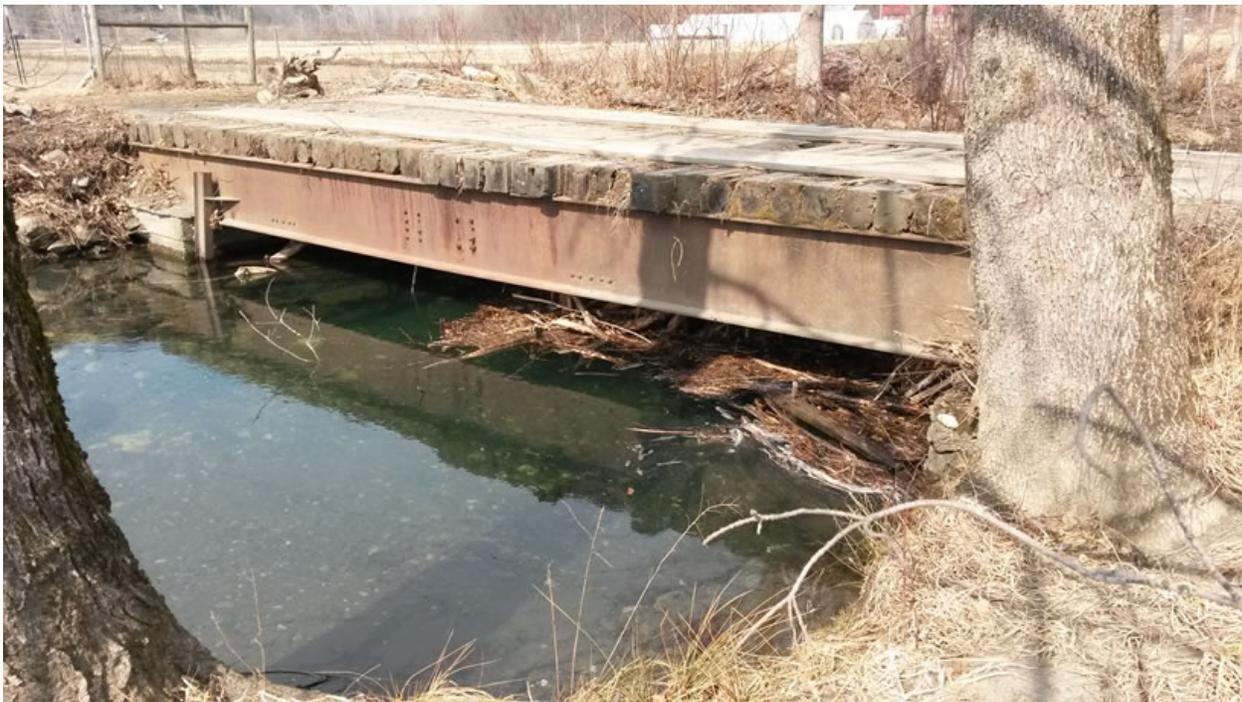
Example of a problem crossing, undersized, that gets clogged with woody debris and causes the stream to flood fields upstream during very high flows.
